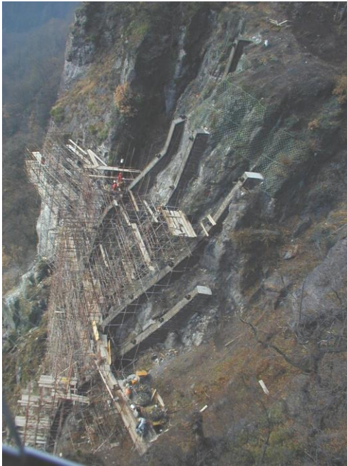
Condino (TN). Volcanic Breccias, stabilization projects of unstable blocks for a height of 50 m.
